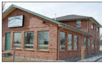
Bernard's Custom Construction Sabott Dental Center • Brighton
